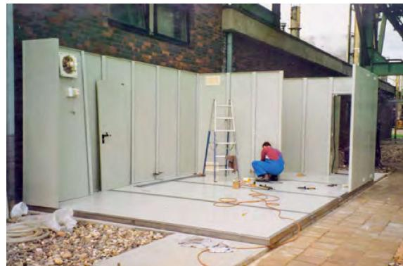
For individual specifications, the width and depth can be flexibly extended in 200 mm increments thanks to our modular system approach.
